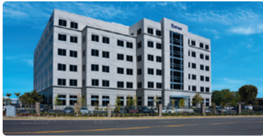
Extron USA West - Worldwide Headquarters
