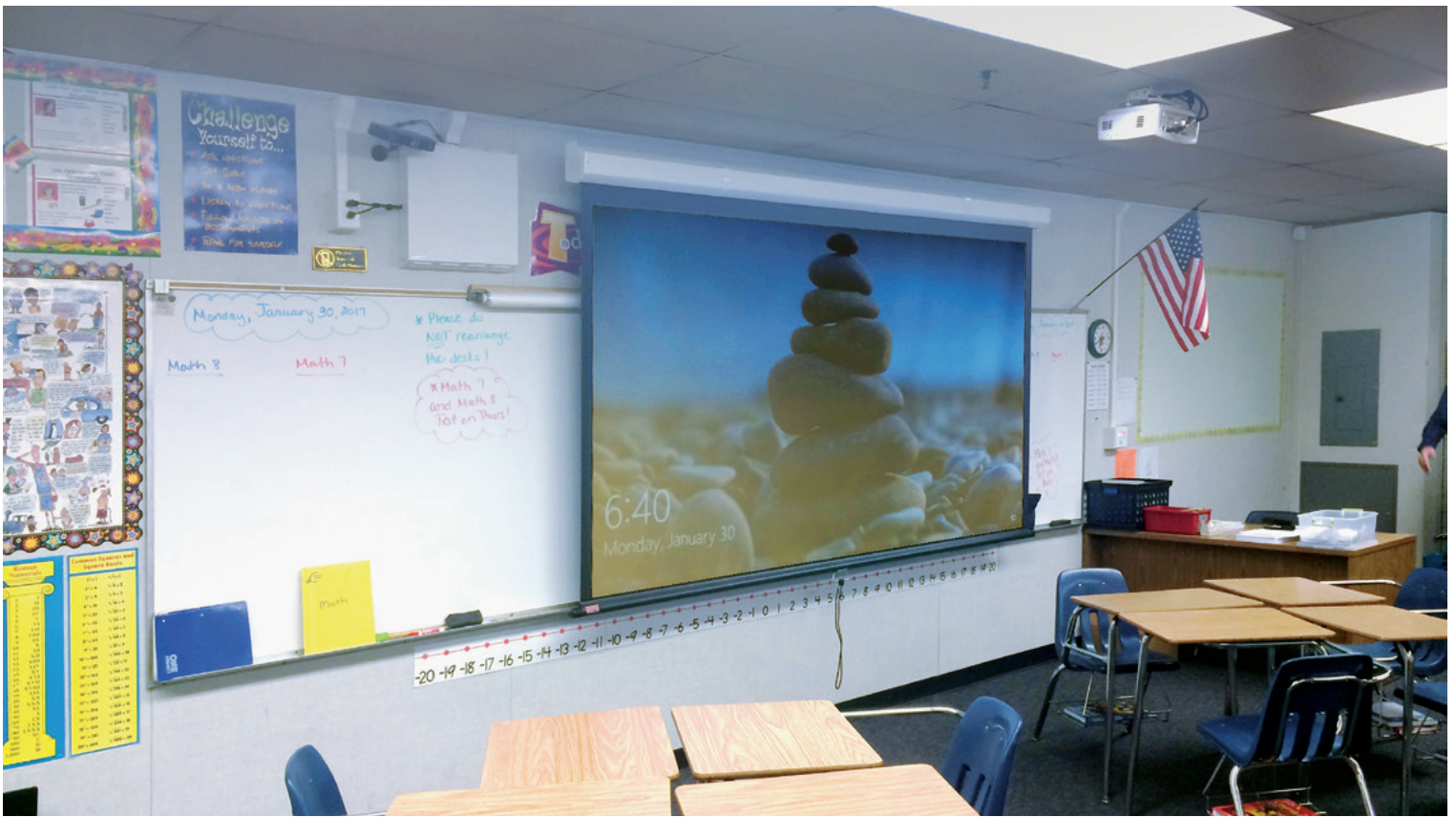
Extron's WallVault Digital System, previously installed in 1,100 rooms as part of a 2014 district-wide campus renovation initiative, is being upgraded at all middle schools and high schools with the Audio Decoding LinkLicense. This allows GVCCS to broadcast bells and PA announcements directly to classroom speakers. Photo courtesy of Murrieta Valley Unified School District.
