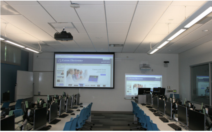
A press on the TouchLinkPro touchpanel's capacitive touchscreen lowers a projection screen in front of or to the side of the whiteboard, depending on room layout.
