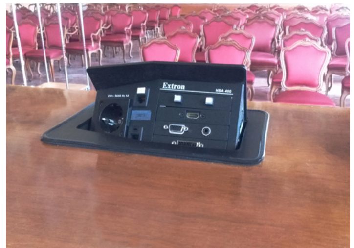
Extron Hideaway HSA 400 units offer AV connectivity and power at the table.
